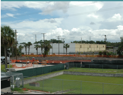
Solar-powered backup power sources were used for the perimeter air monitoring system.
