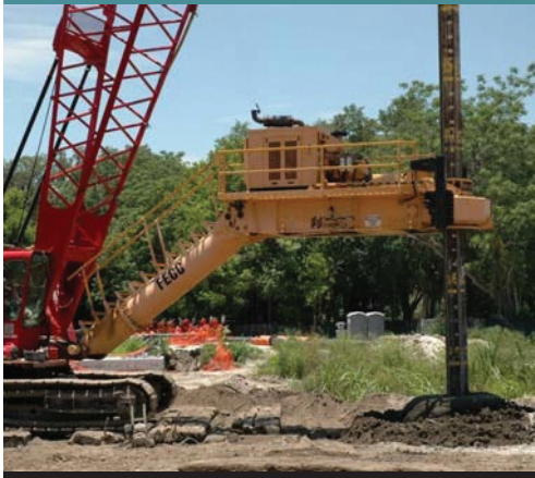
Soil stabilization activities at Sanford Gasification Plant site.
